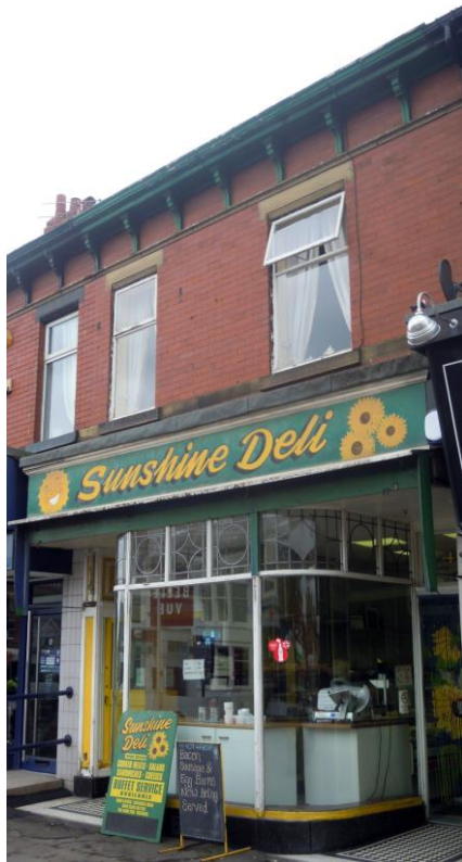
Original shop front - before
